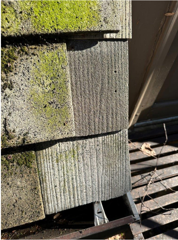
Asbestos shingles
