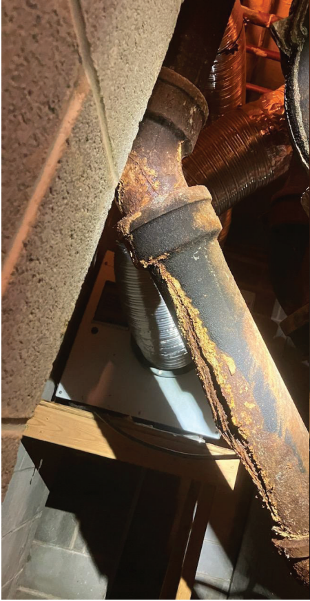
Collapsed Drain Lines
