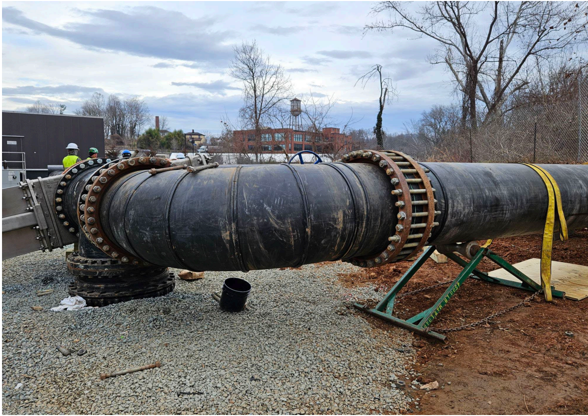
55 million gallons per day pumping bypass system
