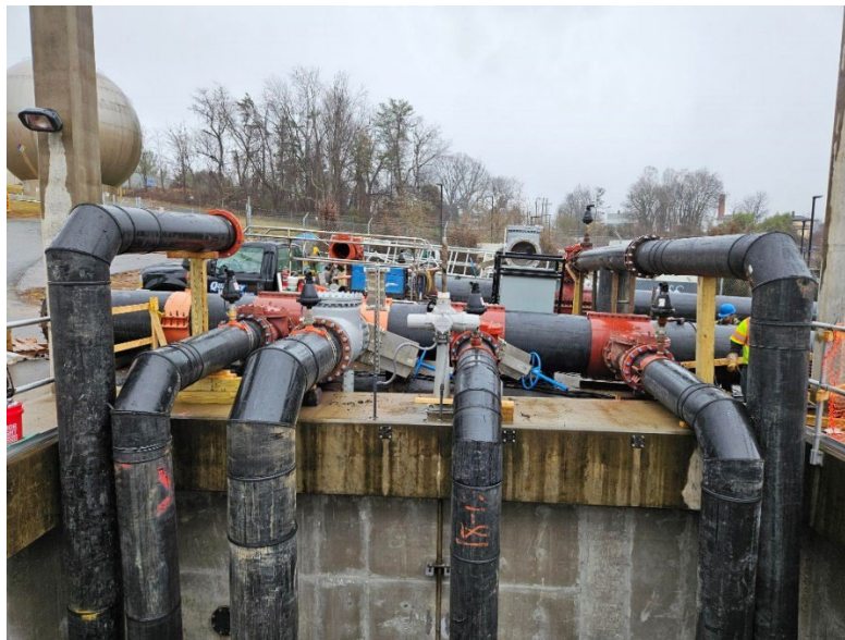
55 million gallons per day bypass pumping system
