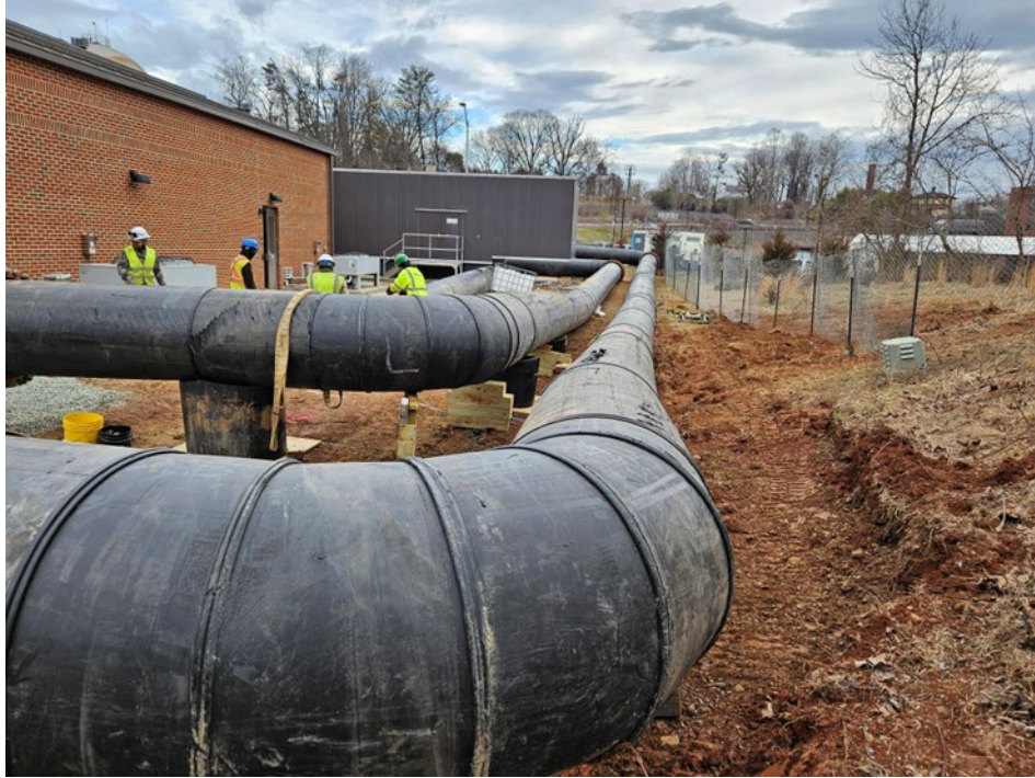
Large bypass system pipes
