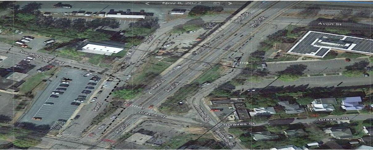
Replacement of structurally deficient bridge with new multi-modal design. A 236 ft bridge crossing BRR/CSX rail lines and Water Street will serve as a gateway into downtown
