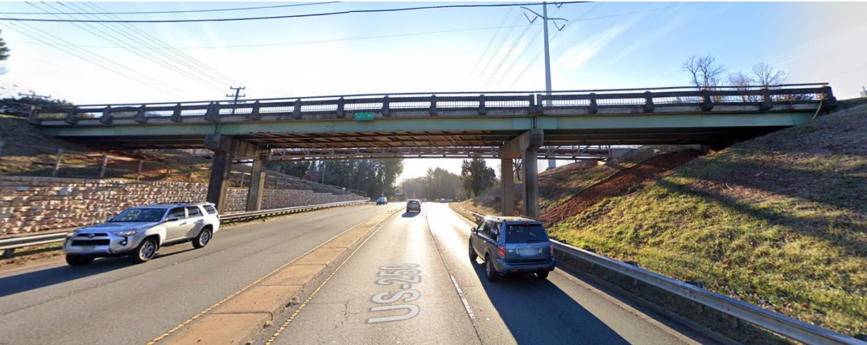
State-of-Good-Repair project replaces the existing two-lane bridge, which does not meet current standards
