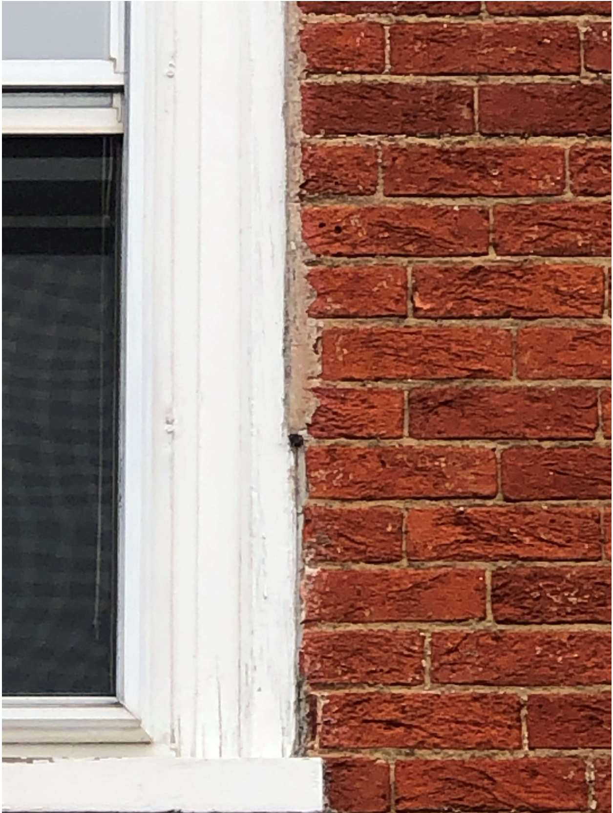
UNORIGINAL WINDOW – NOTE MORTAR AT EDGES
