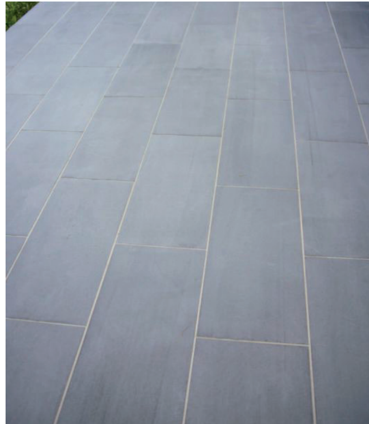
Bluestone w/ staggered joints in running bond pattern
