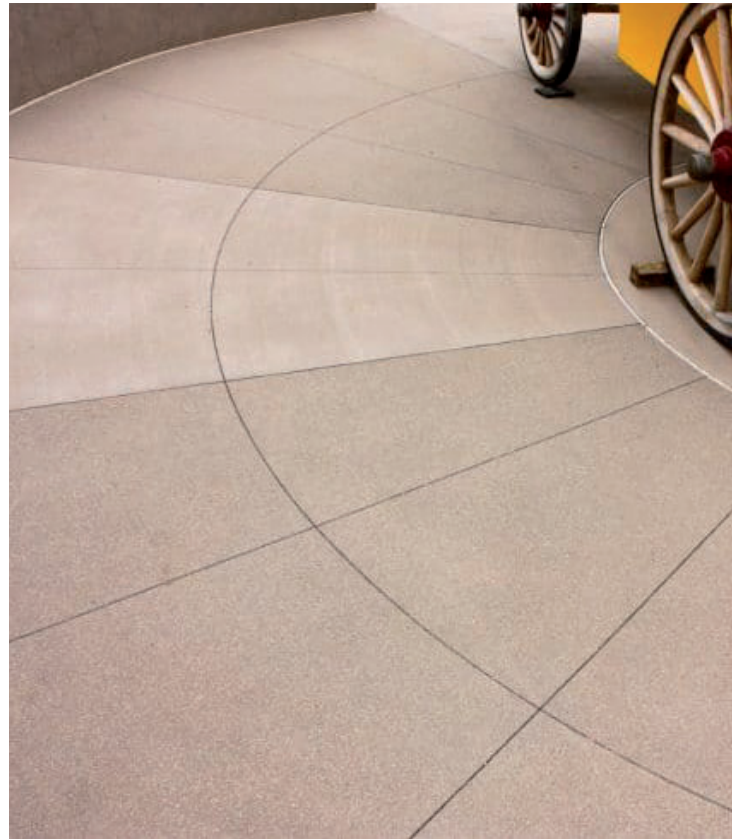
Colored concrete w/ radial saw cut joints
