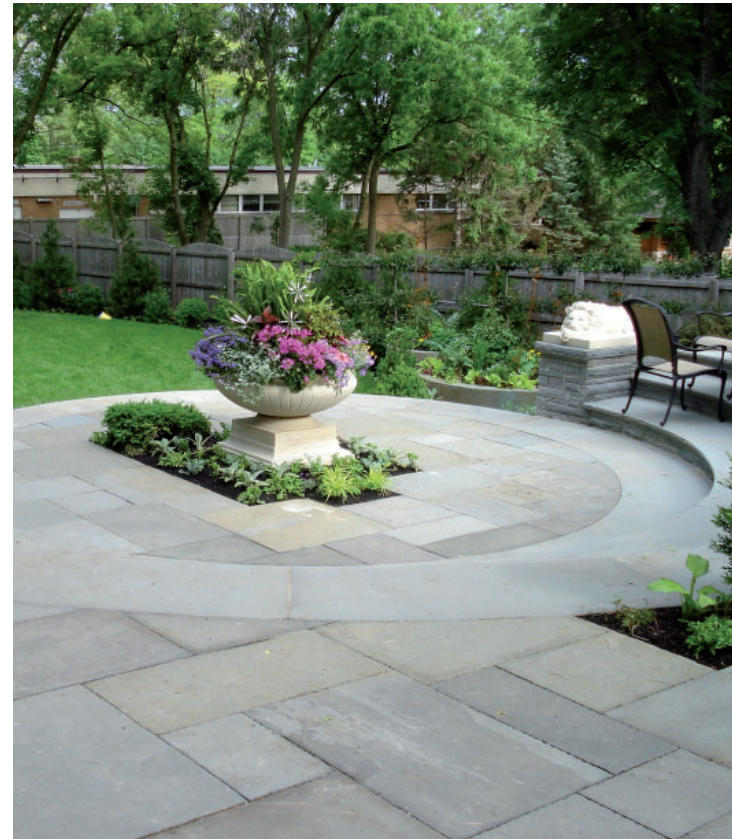
Bluestone pavers combined w/ colored concrete
