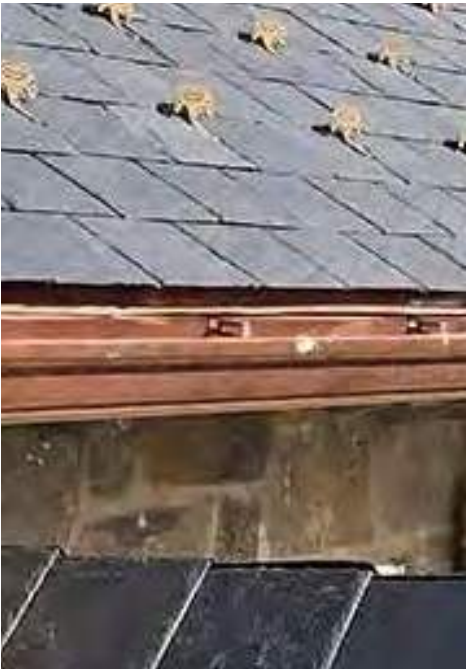
SLATE ROOFING AND COPPER GUTTER
