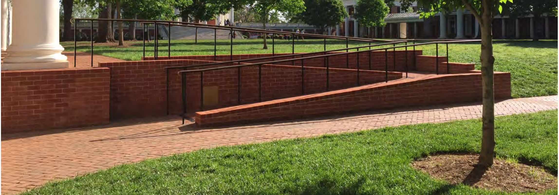
BRICK RAMP AND ORNAMENTAL METAL HANDRAIL
