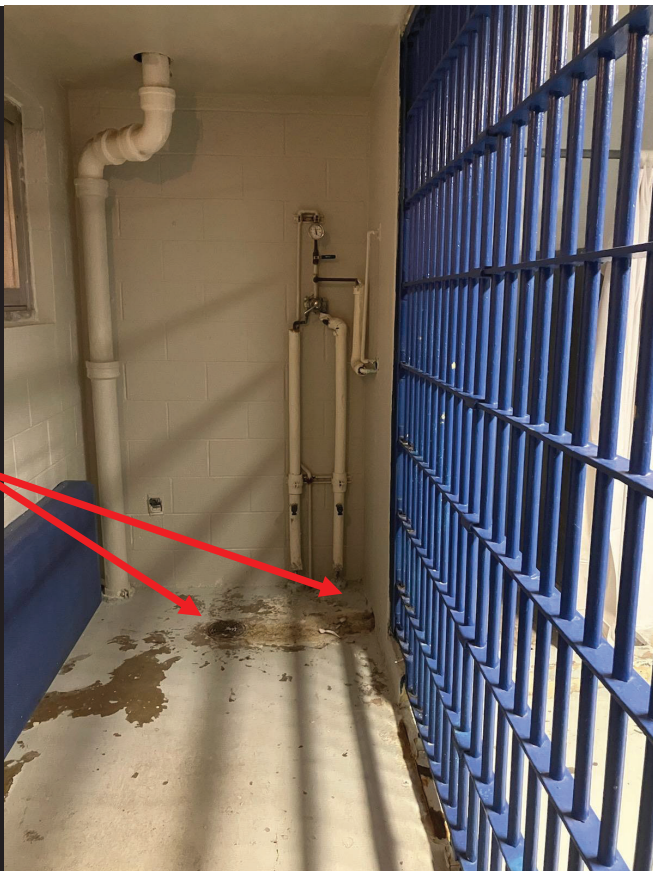
1975 Section Shower Drain runs through opening at bottom of the wall and into drain in the floor
