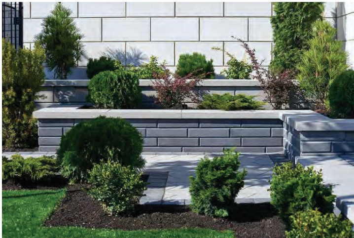
Masonry retaining walls w/ veneer to match the building
