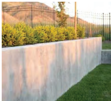
CONCRETE RETAINING WALL (TYPE 1)
