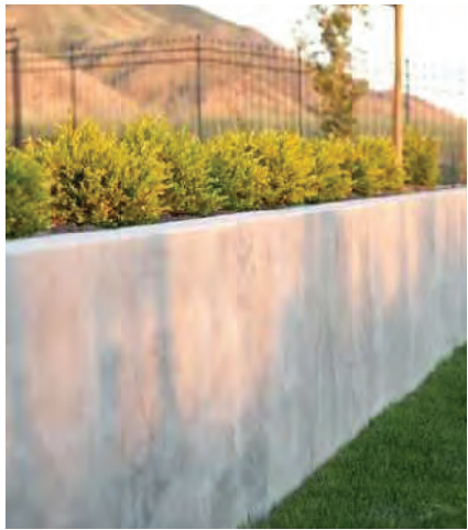
Concrete retaining wall
