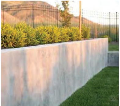
CONCRETE RETAINING WALL (TYPE 1)
