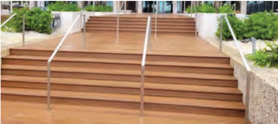
STEPPED TERRACE WALL - CONCRETE WITH WOOD LOOK CLADDING (TYPE 3)
