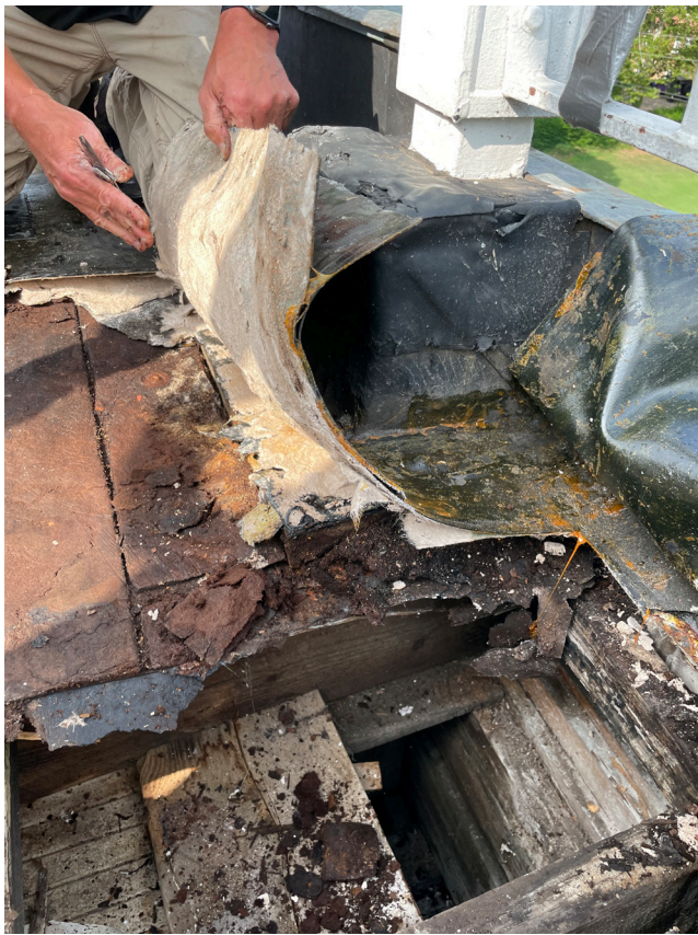
JULY 2022 - DESIGN DEVELOP ASKED TO EVALUATE EXISTING ROOF. DISCOVERED SEVERE DETERIORATION AND DAMAGE TO EXISTING HISTORIC PORTICO
