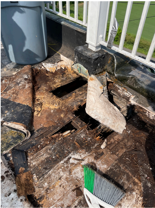
JULY 2022 - DESIGN DEVELOP ASKED TO EVALUATE EXISTING ROOF. DISCOVERED SEVERE DETERIORATION AND DAMAGE TO EXISTING HISTORIC PORTICO
