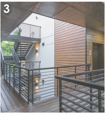
STEEL RAILINGS PAINTED BM163- "MIDNIGHT OIL" WITH WOOD RAILINGS STAINED TO MATCH DECKING
