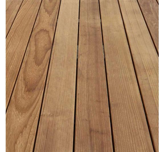
Hardwood decking - black locust, white oak or thermally modified ash finished in multiple clear coats of spar varnish. In the months following installation, the wood will look something like the photo on right. Over time, it will tend to weather to a silvery hue like the photo on the left.
