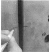
3b Align the proper template lock centerline horizontally with the lock body centerline marked on the frame. Peel the adhesive backing and paste the folded template square to the frame.
