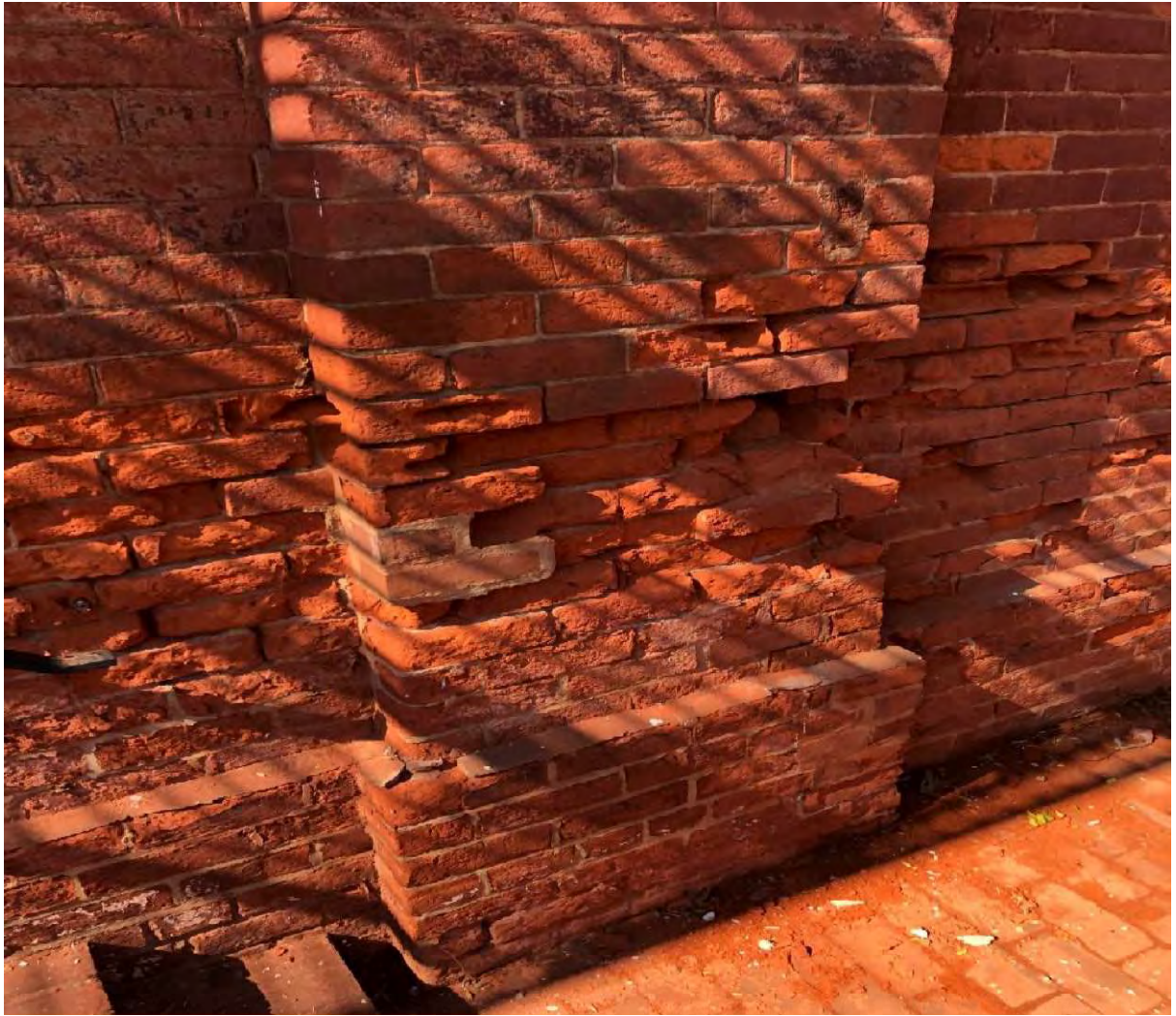
PHOTO 3 – FAILING BRICK CONDITION
