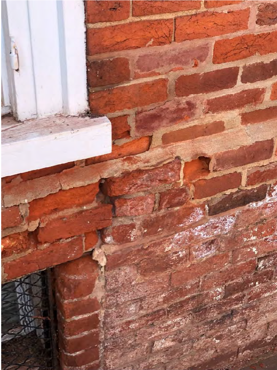
PHOTO 5 – FAILING BRICK
