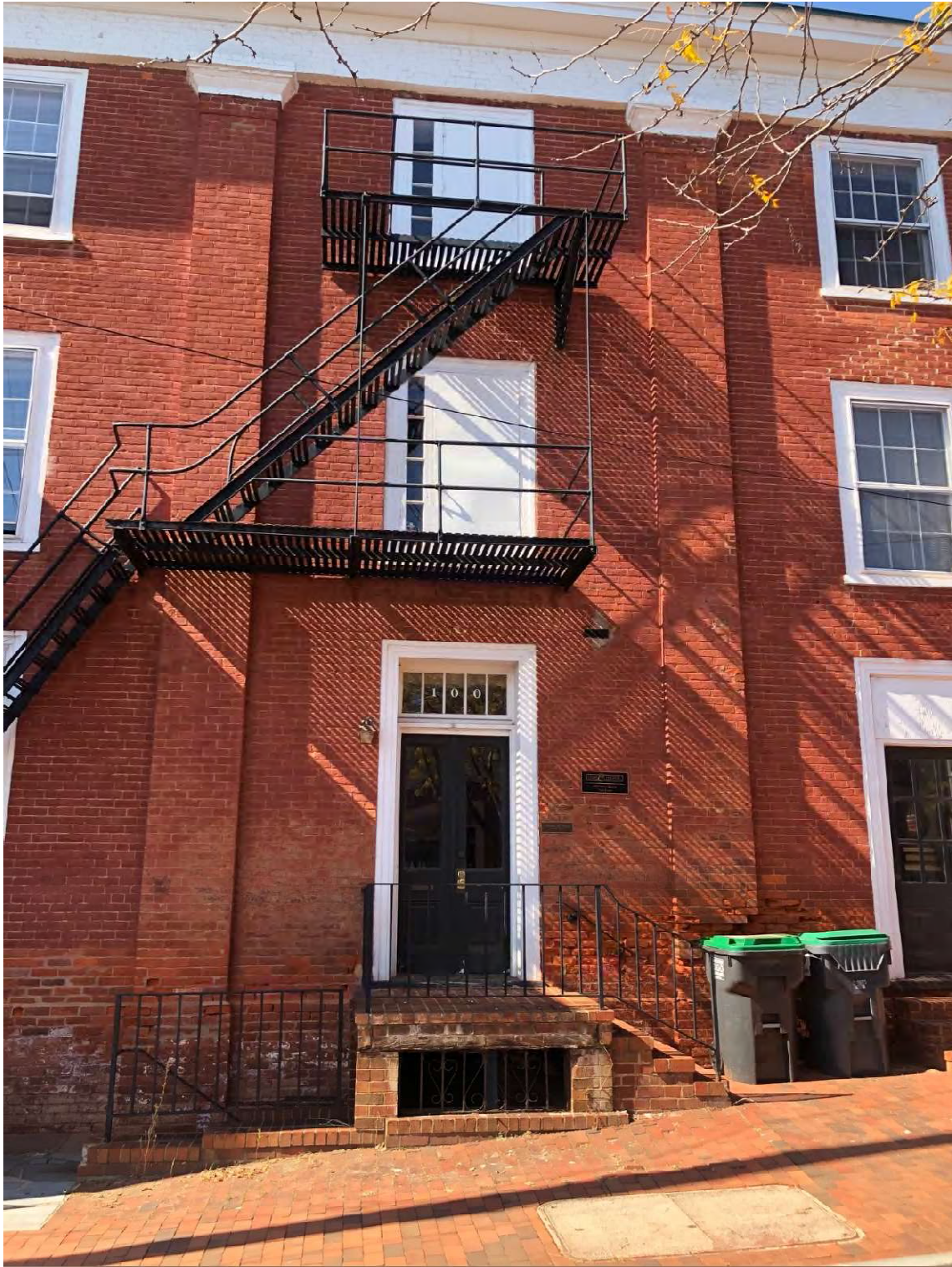
PHOTO 10 – FAILING BRICK AT STREET LEVEL, FIRE ESCAPE TO BE WRAPPED BY PORTICO
