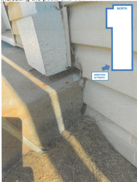
Photo 1: Imprints of the post in concrete indicate the slabs original position.
