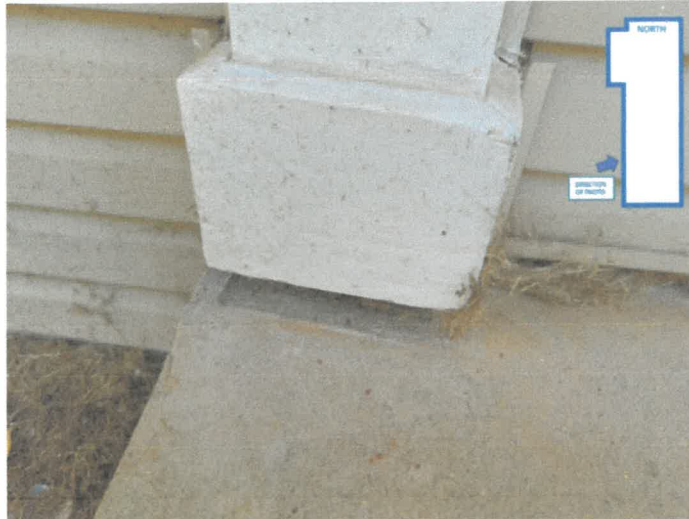
Photo 2: Imprints of the post in concrete indicate the slabs original position.
