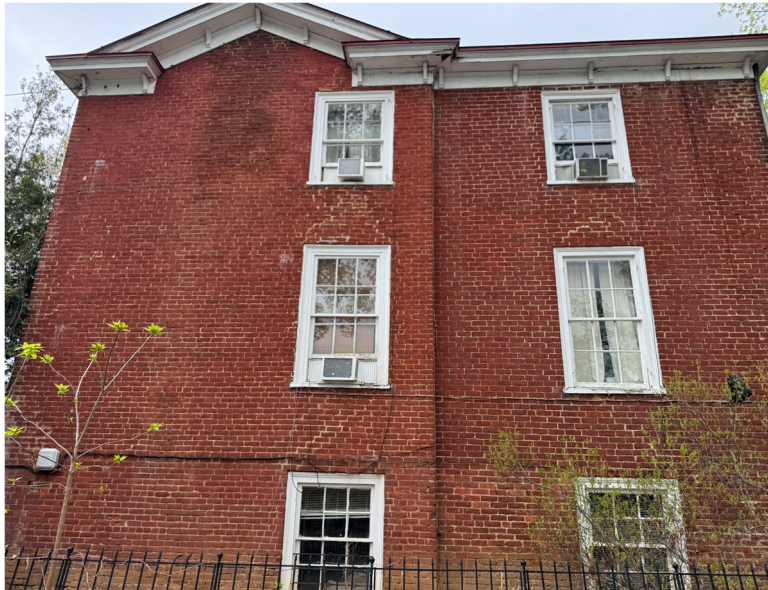
Photo 3: East side of the building with some warping of the window frame and evidence of previously older repair to the brick under the windows.
