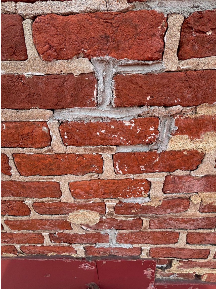
Mortar Detail & Repairs
