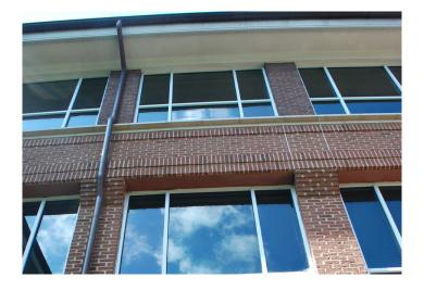
**Copper Gutters & Downspouts - Half Round**To Match Existing
