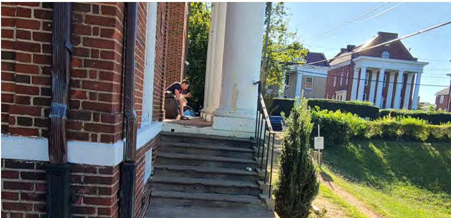
LEFT SIDE EXTERIOR STAIRS - DETERIORATION TO CONCRETE AND BRICK & PREVIOUS ATTEMPTS AT REPAIR
