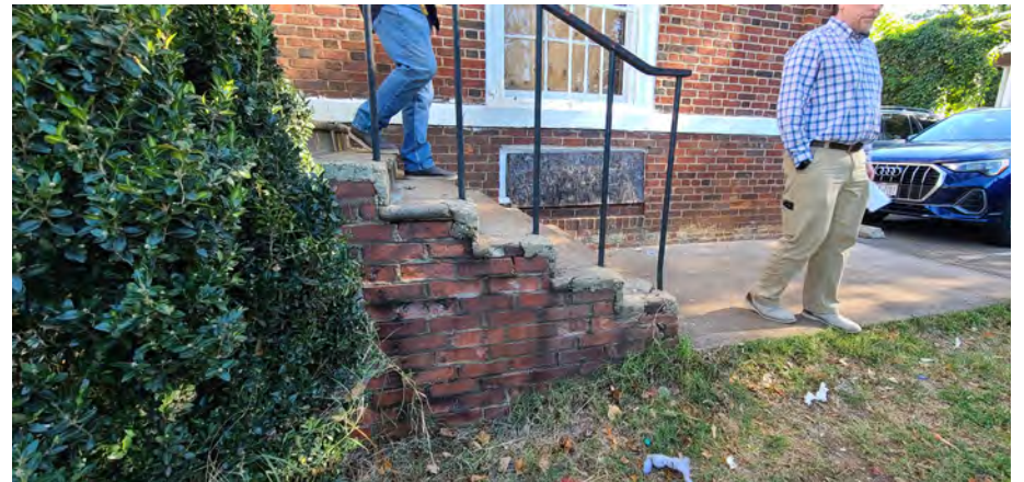
RIGHT SIDE EXTERIOR STAIRS - DETERIORATION TO CONCRETE AND BRICK & PREVIOUS ATTEMPTS AT REPAIR
