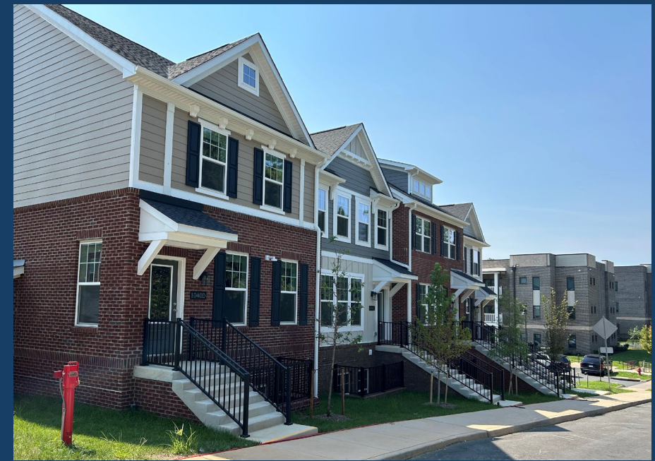
South First Street Phase 2
